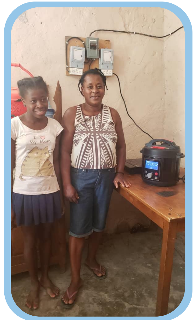
Haitian family with their new electric cooking installation
